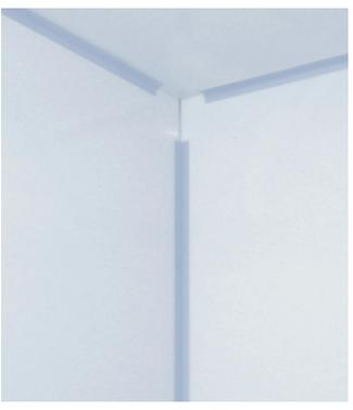
**1.** The vinyl anchor strip is affixed into the corners around the ceiling perimeters and the inside corner(s) of the walls.
