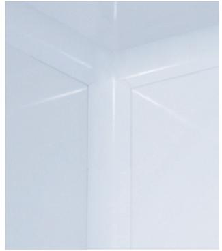
**3.** The field cut-to-fit straight lengths of coving snap securely into place.
