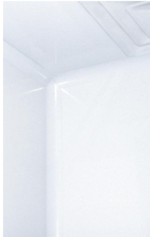
Eliminating 90-degree corners with CleanCove helps assure that your cGMP facility will be validatable. CleanCove is compatible with new construction or retrofit applications, easily upgrading existing facilities to cGMP compliance.
