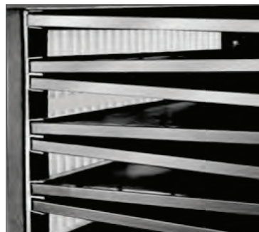
Side Access Carbon, side view, showing "V" bank trays.
